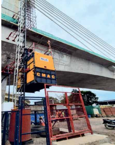
PM Hoist for Cable Stayed bridge
