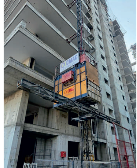
PM Hoist with Rebar Carrier
