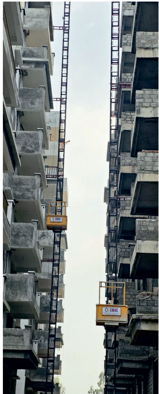
Standard-MFH Multi Functional Hoist -110 mtrs
