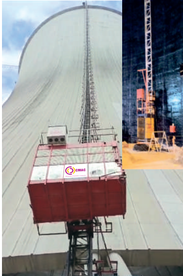
Curved Hoist for NDCT & Inclined hoist for Chimney
