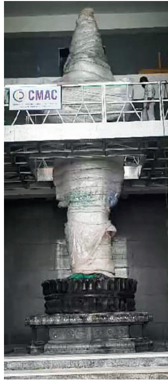
Access Suspended Platform @ Vijayakeeladri Temple Vijayawada, AP
