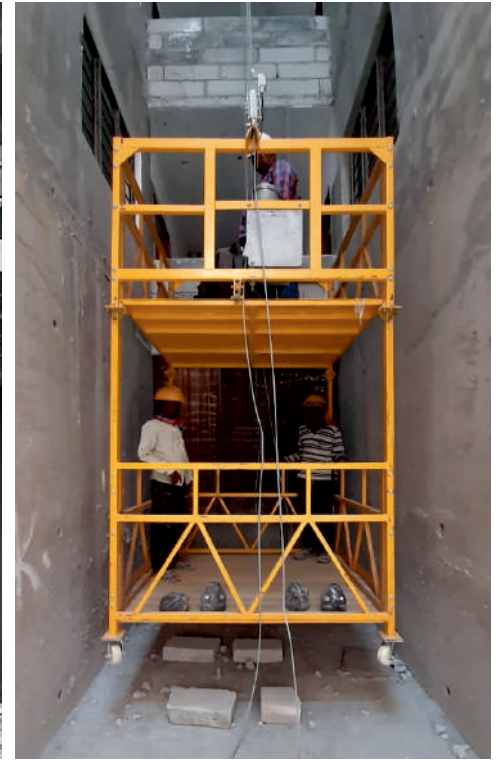
Special Double Decker SRP for Lift Shaft
