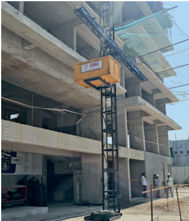
Multi Functional Hoist (MFH)-CMAC Rambo with Rebar Carrier
