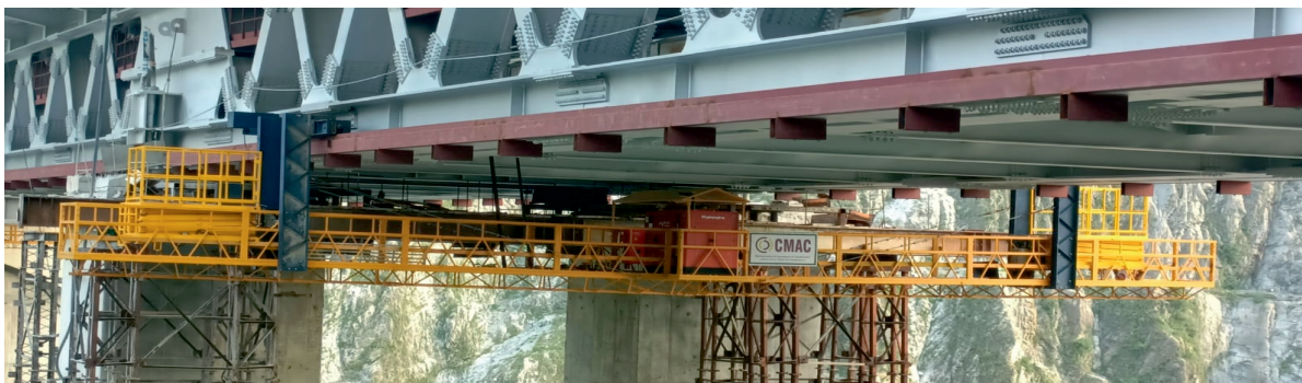
Self Propelling Maintenance Platform @ 331 Meters Height Horizontal Travel (290 Meters, 70 Meters, 80 Meters) Anji Khad River @ Jammu, First Cable -Stayed Railway Bridge in India
