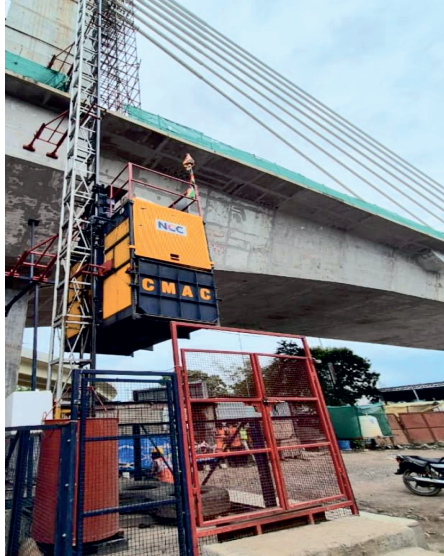
PMH for Cable Stayed bridge
