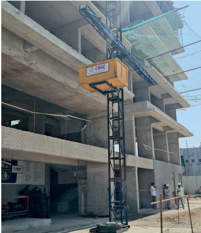
MFH-CMAC Rambo with Rebar Carrier
