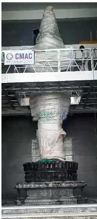
Access Suspended Platform @ Vijayakeeladri Temple Vijayawada, AP
