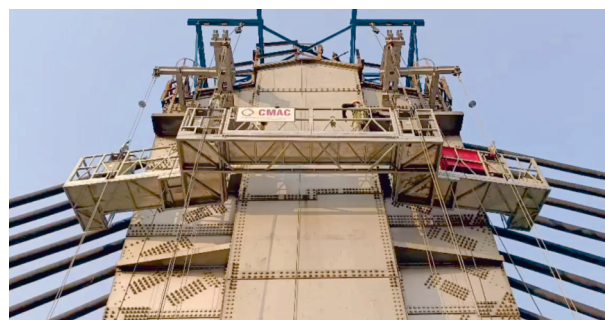
Varying electro mechanical access platform @ Vidyasagar Setu, Kolkata
