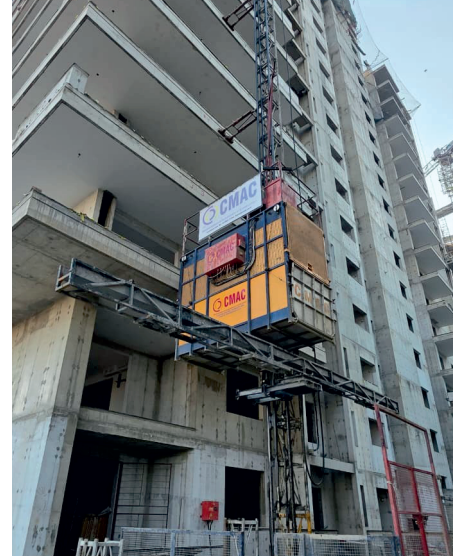
PMH with Rebar Carrier
